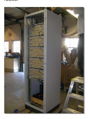
In this case its 20 radios and 20 Network Interfaces in one rack. Power and UPS at the bottom and LAN switches at the top.
